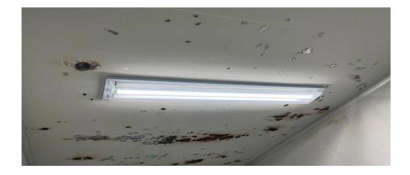
Chemically damaged panel - rough, discolored surface with cracks
